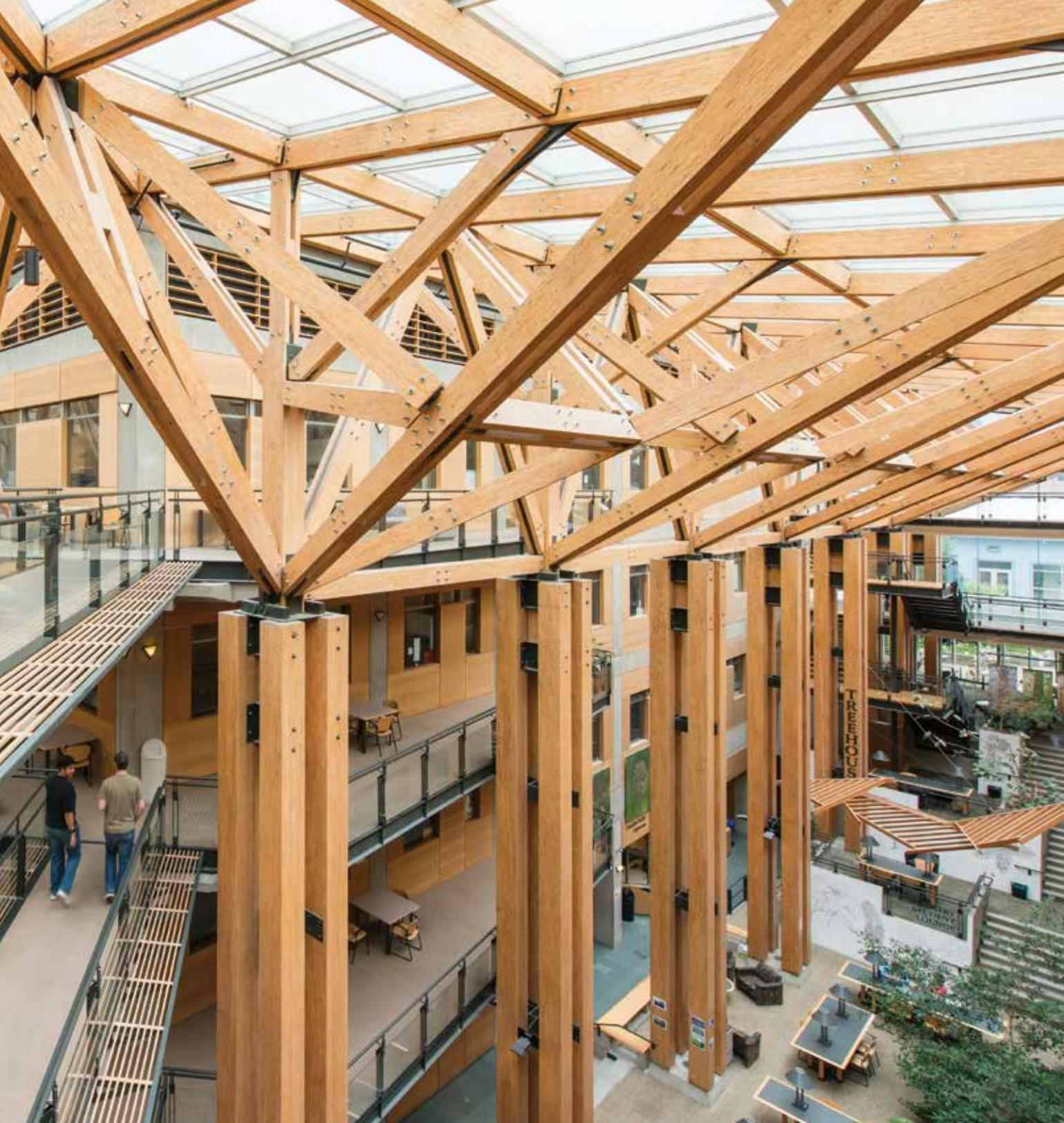
*The Forest Sciences Centre, completed in 1998 at UBC, integrated wood construction throughout the building to showcase wood as both a structural and aesthetic material. To achieve compliance with the prescriptive building code requirements of the time, code consultants utilized two primary concepts: the enclosed space and the combustible construction equivalencies.*
