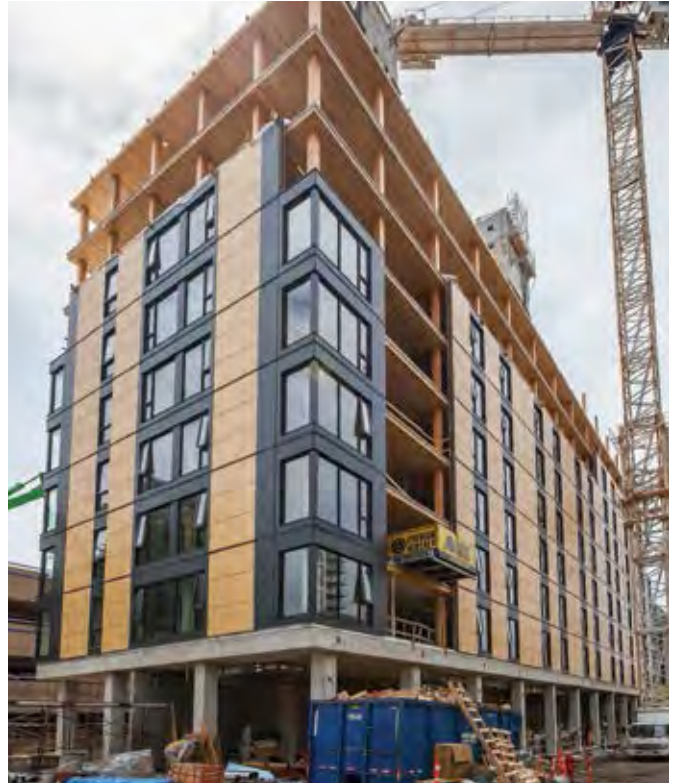
Brock Commons Phase 1 Student Residence is an innovative mass timber hybrid structure at the UBC. Image of construction progress July 2016. Photo Credit: KK Law
