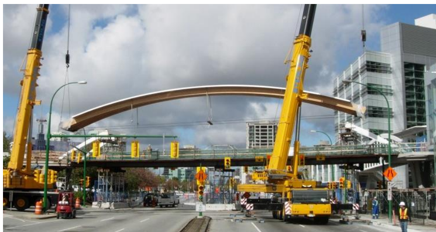
Kingsway Bridge, Burnaby, BC. Spanning 145 feet across a major arterial roadway, Kingsway Pedestrian Bridge's one-of-a-kind construction consists of a timber-steel arch with the post-tensioned segmental precast concrete walkway acting as tension tie.
