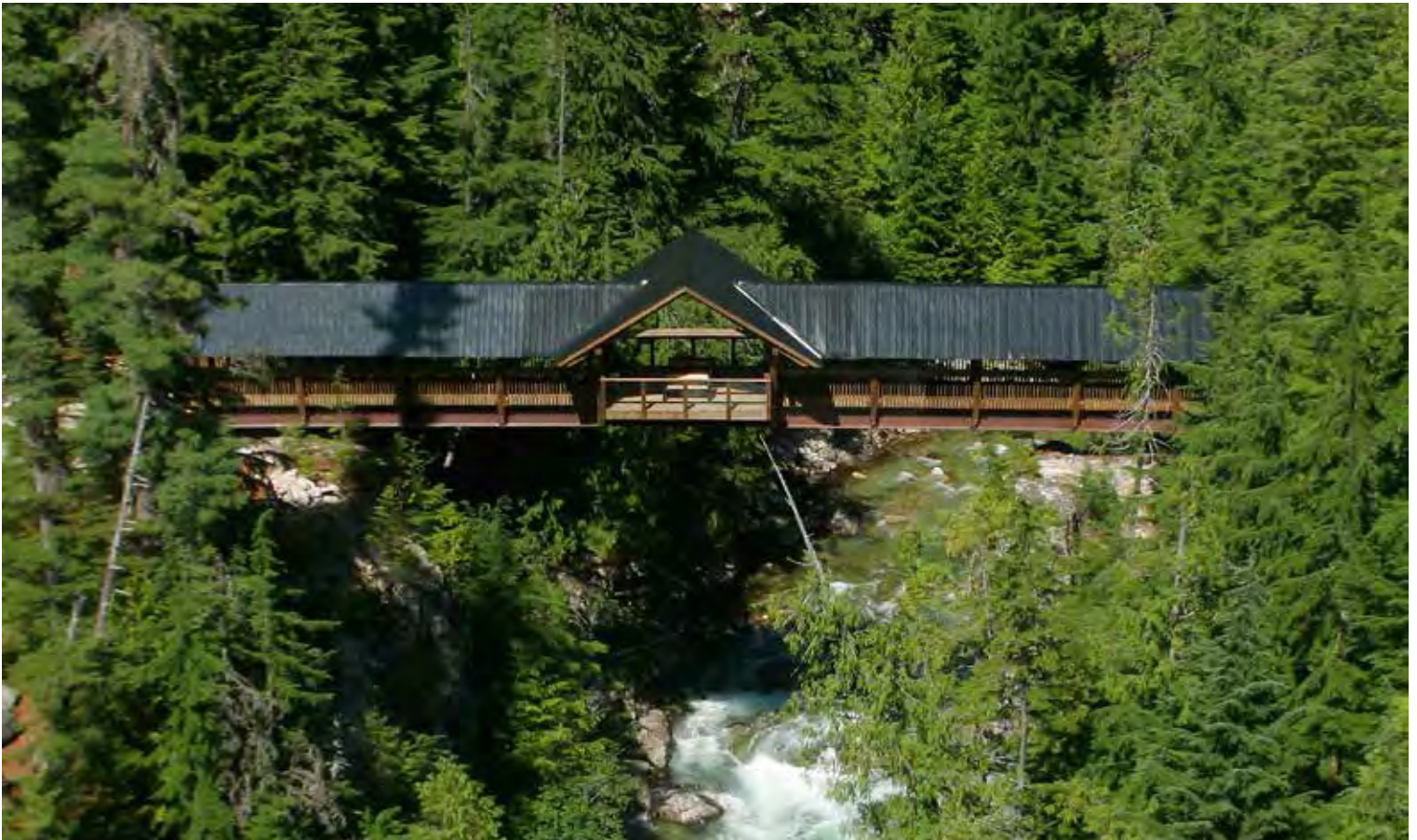
Photo courtesy of Rory McLeod, courtesy of Madden Timber Construction
