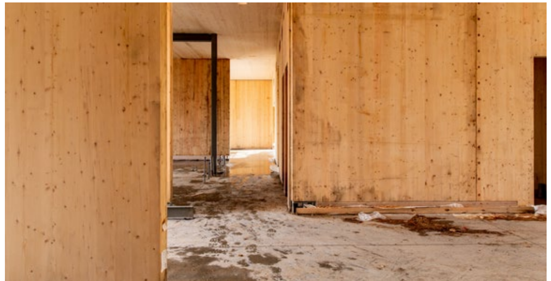
wəkwʌnəs tə syaqwəm Elementary School | Vancouver, B.C. The CLT structure, erected early in construction, needed to be protected from damage and exposure to moisture. (HCMA, 2009)
