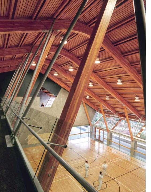
"The materials for the building were chosen to align with the architectural, structural and mechanical requirements. The exposed glulam beams are aesthetically pleasing while spanning significant distances. The prefabricated, architecturally expressed wood panels perform multiple functions, being integrated with the building ventilation system, while spanning between the glulam purlins and acting as part of the roof diaphragm."
