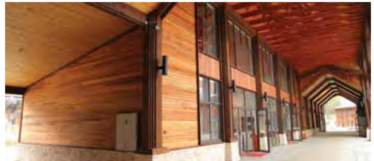
The building incorporates standard dimension framing lumber and oriented strand board sheathing, with western red cedar cladding used on the exterior.
