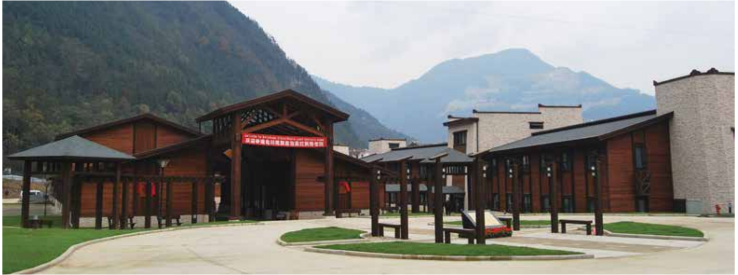
The facility will help demonstrate the technology for multi-storey, multi-residential accommodation specially designed for the elderly population.
