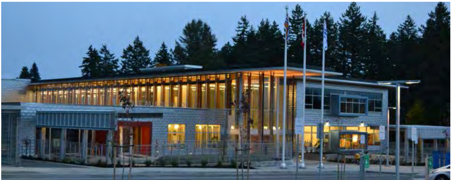
Photo courtesy of McFarland Marceau Architects
