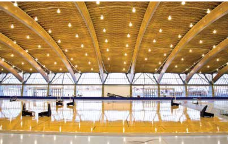
Above: The Richmond Olympic Oval showcases the ingenuity and innovation of B.C. wood products with a massive wood wave roof encompassing 6.5 acres. Photo: KK Law
