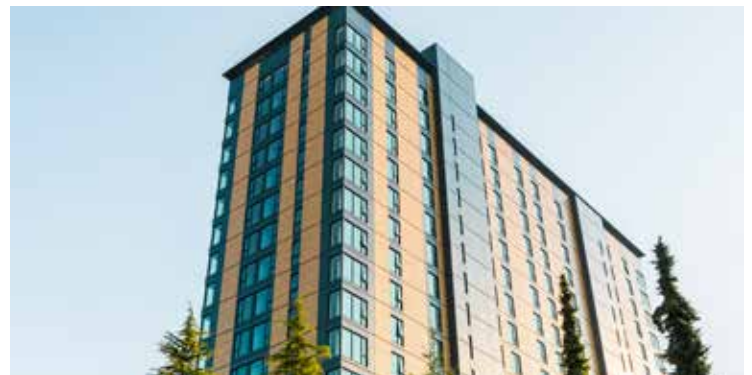
Brock Commons Tallwood House | Architect: Acton Ostry Architects Inc. | Photo: Brudner
