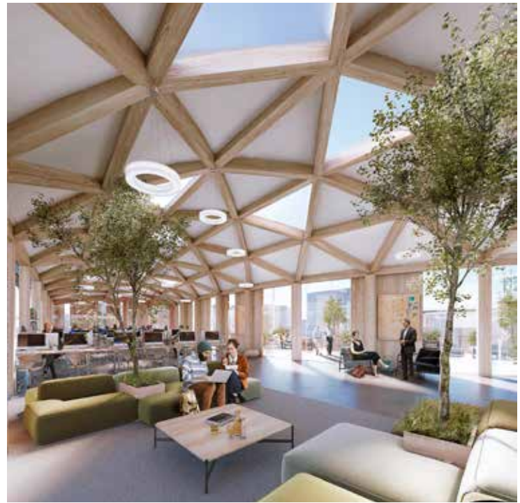
Office interior will feature a glulam ceiling.
