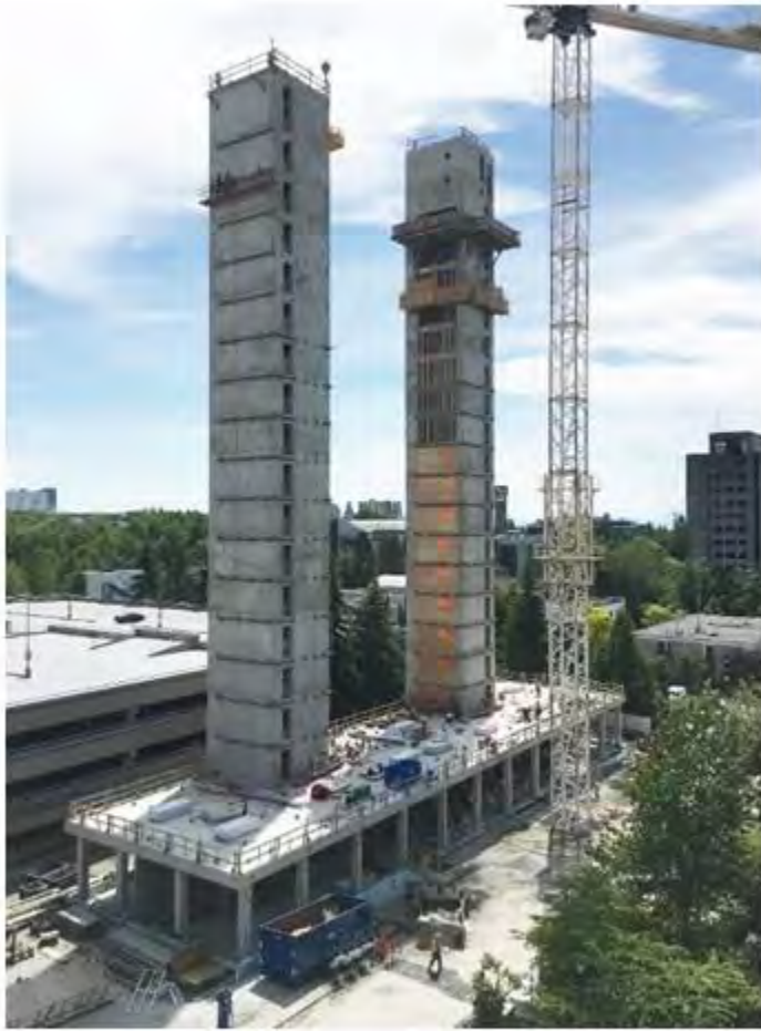
Concrete cores + slabs
