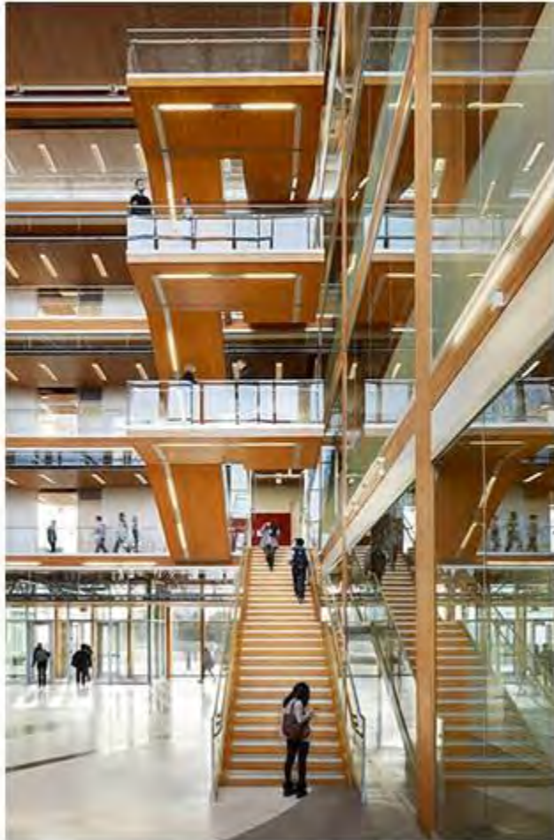
UBC Earth Sciences Building | 6 storeys Vancouver, Canada
