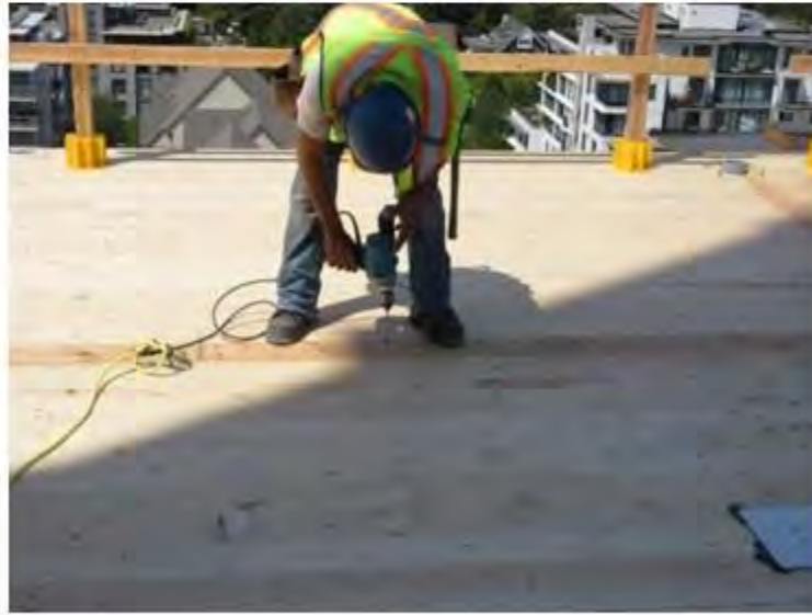
Plywood splines
