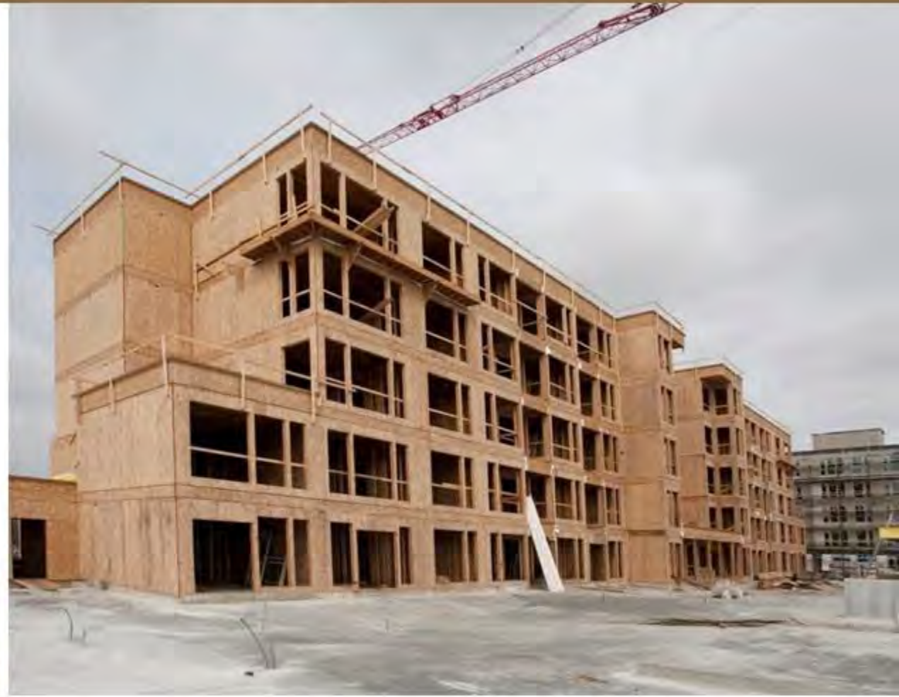
Typical British Columbia Mid-rise “stick-built” or wood-framed construction
