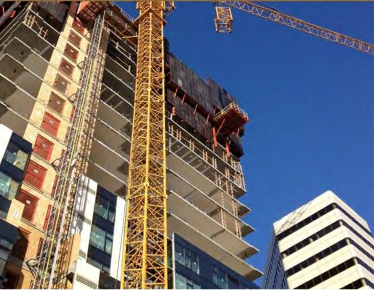
Typical British Columbia High-Rise cast-in-place reinforced concrete
