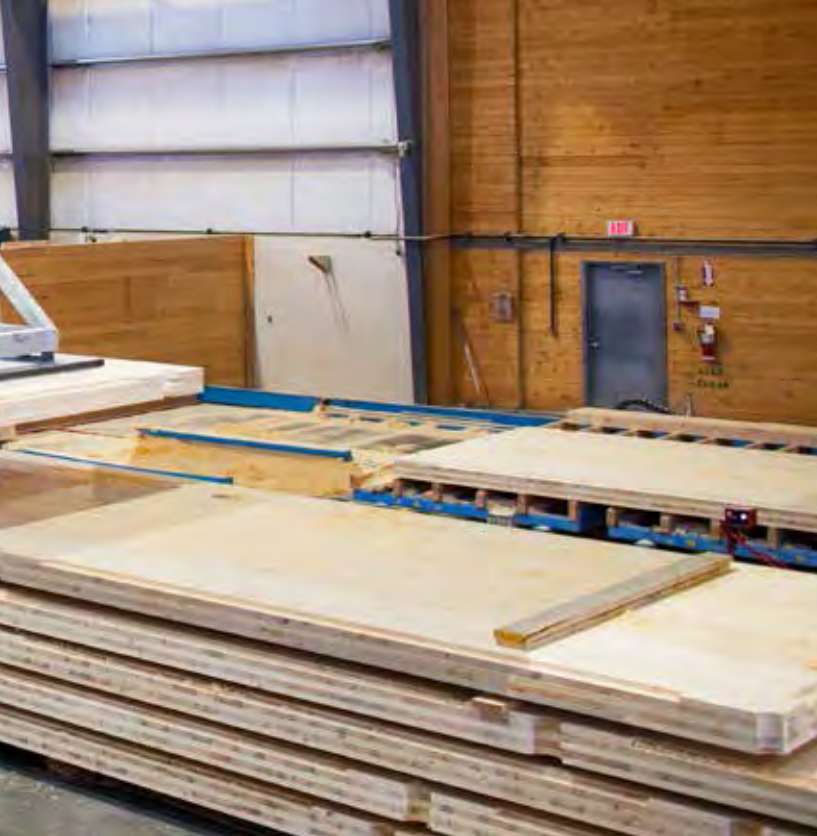
Assembly of Brock Commons CLT panels. Photo courtesy of Brudder
