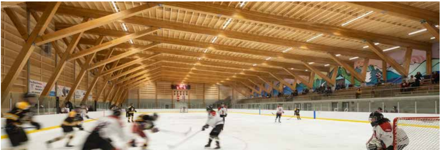
Photo: Ema Peter Photography, courtesy Hemsworth Architecture
