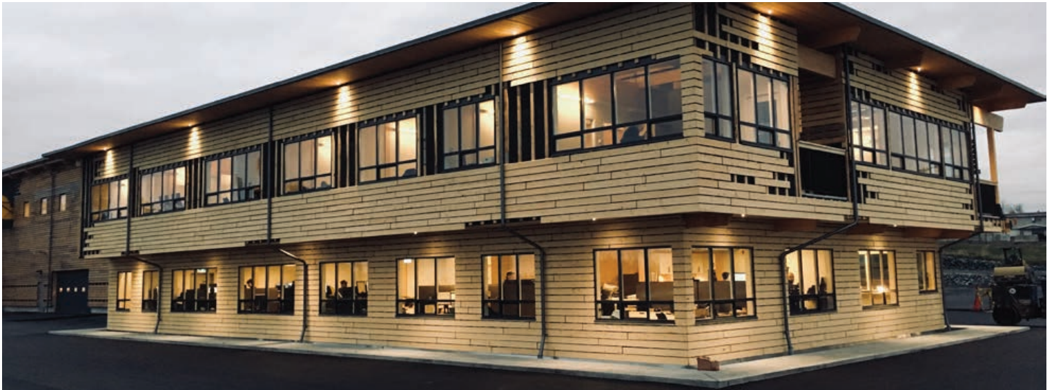
Photo courtesy of StructureCraft Builders.
