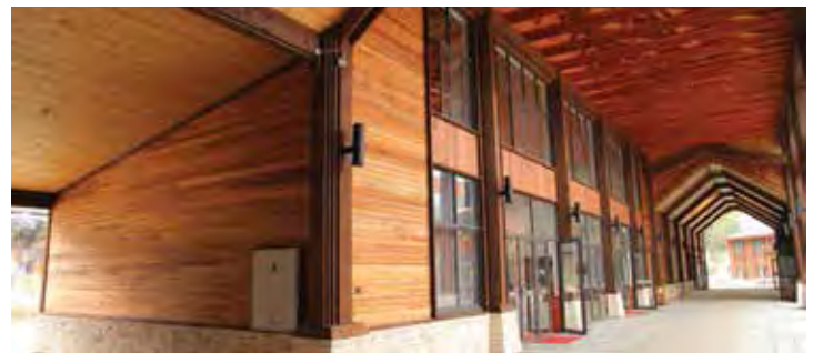
The building incorporates standard dimension framing lumber and oriented strand board sheathing, with western red cedar cladding used on the exterior.
