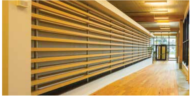
Reflecting its commitment to sustainability and to create a healthy and inspiring workplace for its employees, Mountain Equipment Co-op chose B.C. wood products as the primary building material for its new Vancouver, B.C.-based headquarters. An exposed glulam post and beam system comprise the primary structure and the floors were constructed using NLT panels. Photo: KK Law
