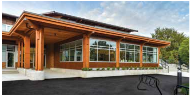
As part of the Province of B.C.'s seismic mitigation program for schools, J.W. Sexsmith Elementary was constructed almost entirely of B.C. wood, incorporating species such as Douglas fir, spruce and western red cedar. The result is a structure built to withstand seismic events, complemented by wood finishes which create a warm learning environment. Photo: courtesy of Iredale Group Architecture
