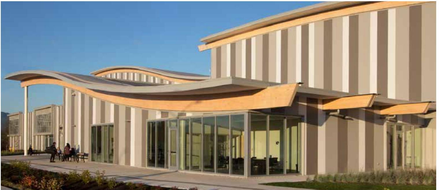
*“It was important for us to build an iconic building that the City of Surrey would be proud of. Most arena buildings are built with steel or concrete which look and feel cold, but this project, with its wood roof deck and structural glulam trusses, gives visitors a warmer experience. We were trying to make this more than just an ice arena, and with the switch from a metal to a wood roof deck, we got a better building.”*
