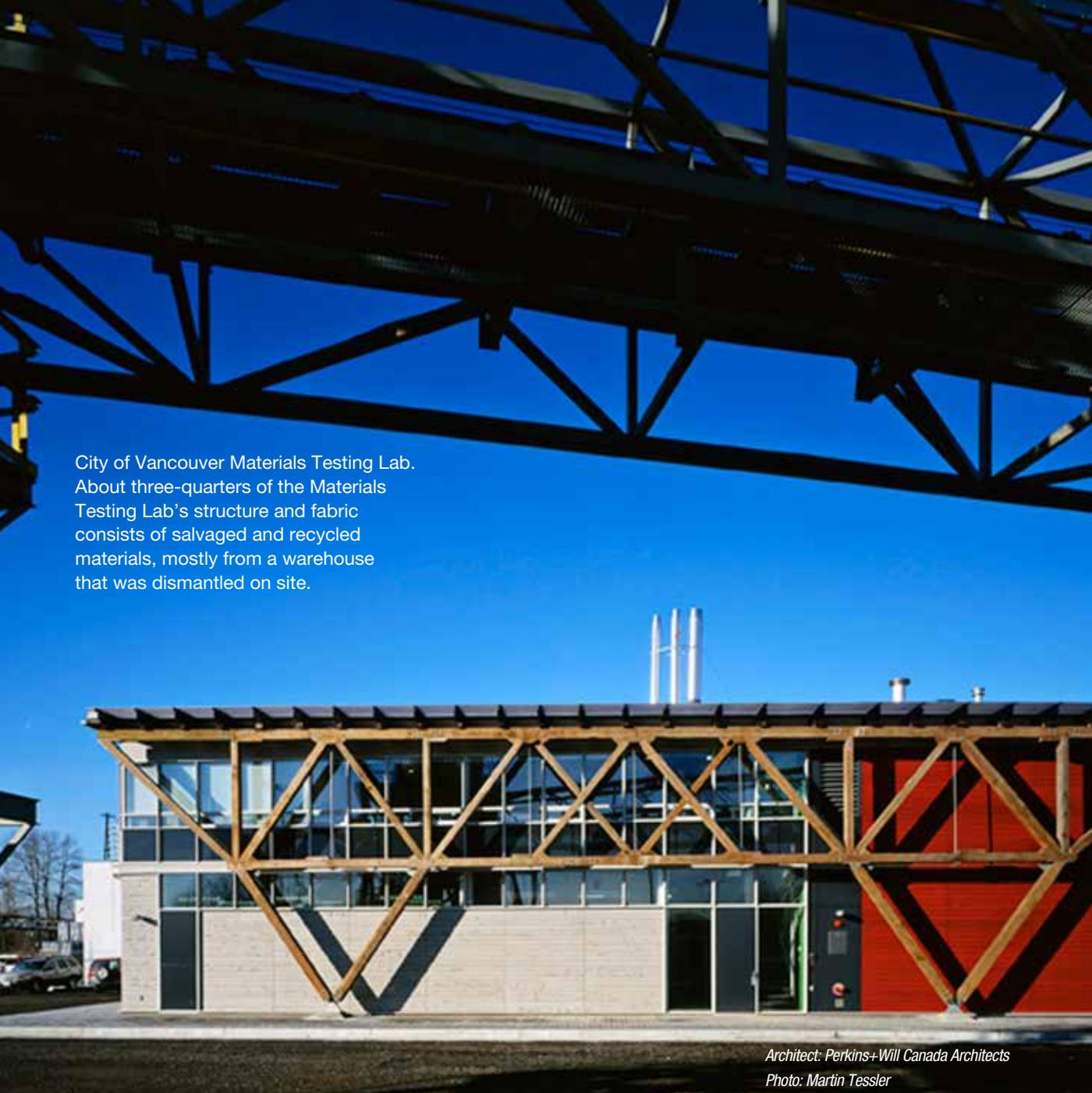
City of Vancouver Materials Testing Lab. About three-quarters of the Materials Testing Lab's structure and fabric consists of salvaged and recycled materials, mostly from a warehouse that was dismantled on site.
