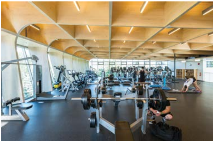
UBCO Fitness and Wellness Centre's egg-crate CLT structure is both lightweight and strong, inspired by the wing structure of balsa wood airplanes. Photo courtesy of Don Erhardt.
