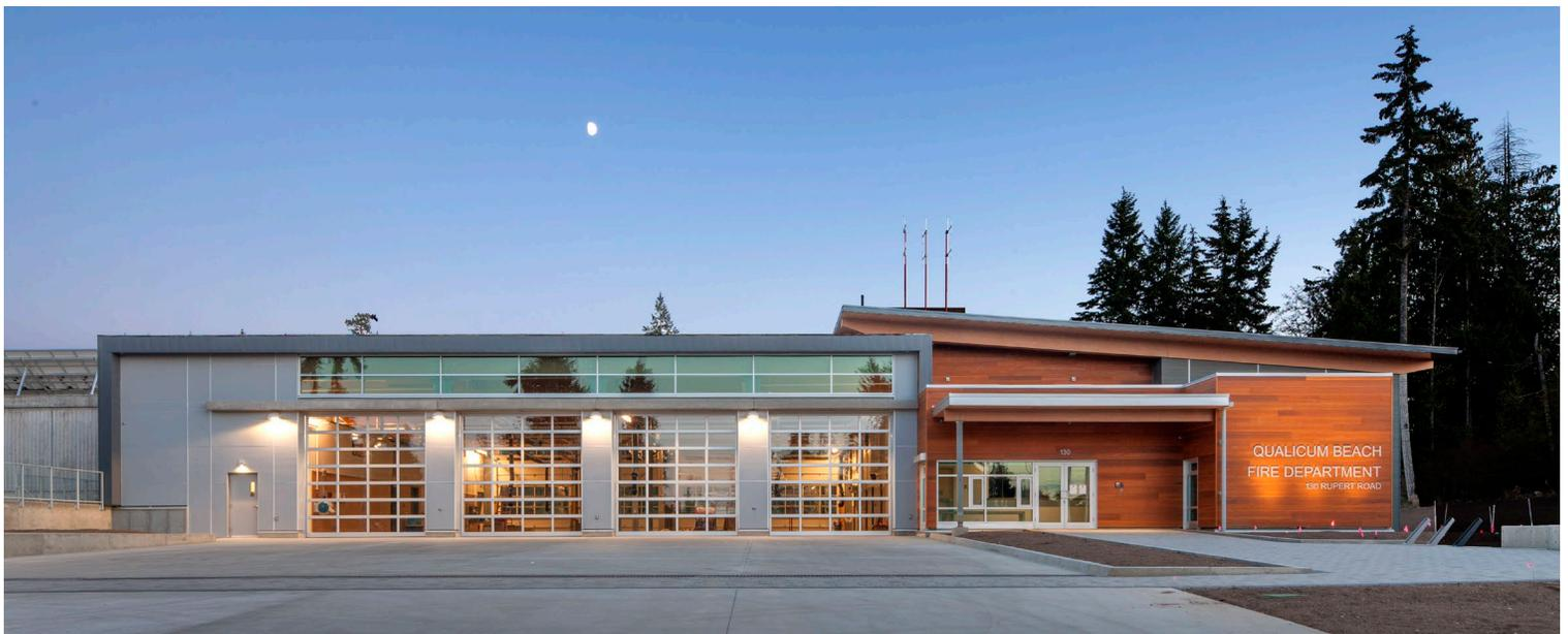
*“The use of solid mass timber panels is an effective option for institutional buildings considering sustainability and performance. Speed of construction is also advanced through the use of prefabricated wood panels. With the Qualicum Beach Fire Hall, the roof panels were erected in only seven days allowing for the roof membrane to be installed much earlier in the construction process.”*
