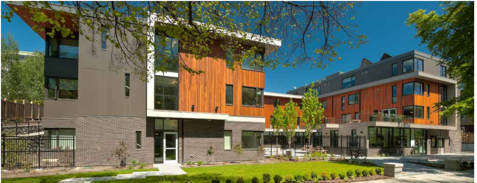
Photo by Destrube Photography, courtesy of Chow Low Hammond Architects
