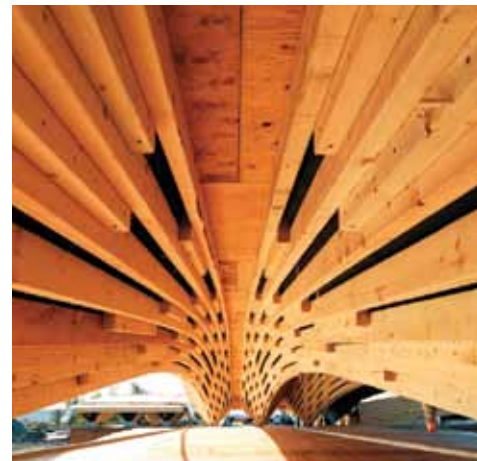
In Richmond, British Columbia, the Olympic Oval's 6-acre (2.4-ha) roof is built with pine beetle wood.
