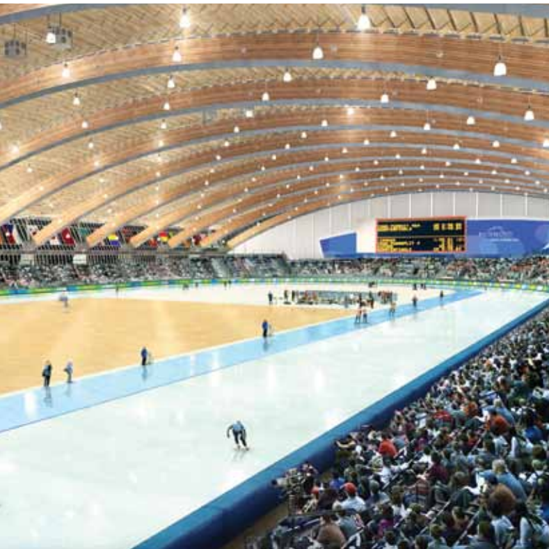
Left image: Richmond Olympic Oval Architect: Cannon Design The venue was built for the 2010 Olympic and Paralympic Winter Games in Vancouver, and is now a multi-sport and wellness facility for the local community. The unique roof system is made with wood affected by the mountain pine beetle infestation in British Columbia's interior, making it an important tool in mitigating the impacts of climate change by sequestering carbon.
